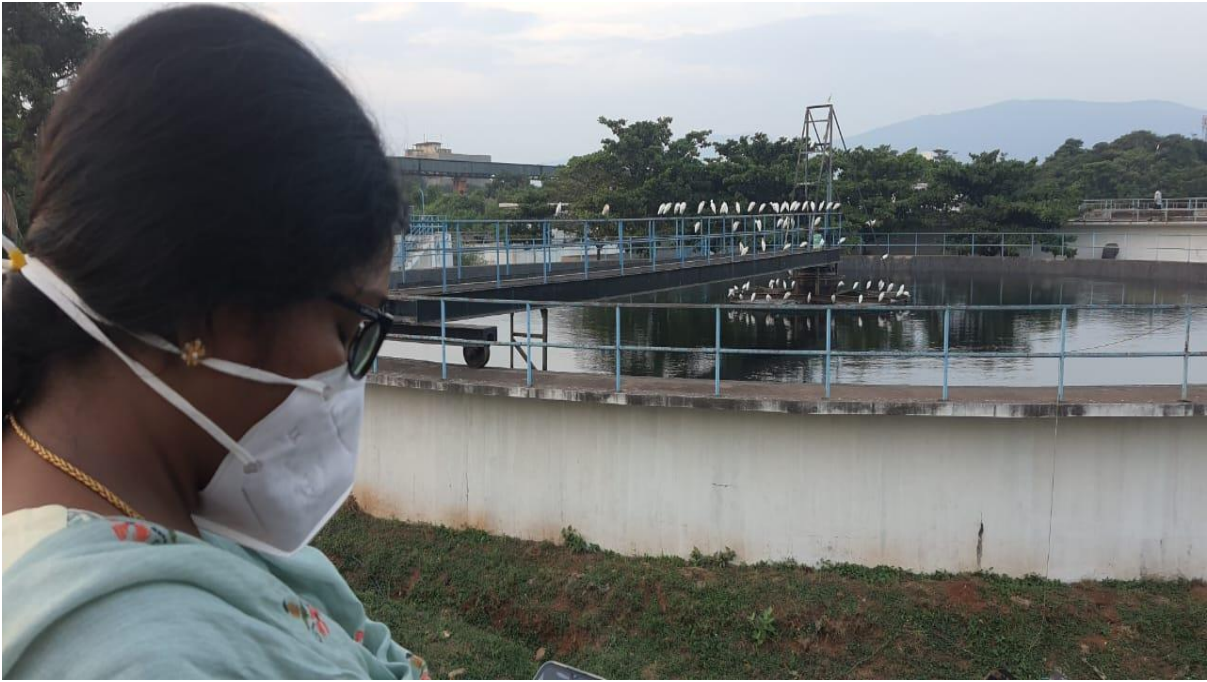
Inspection of 38 MLD, STP at Old Lakshmi Talkies, near Town Kotha Kota Road, Visakhapatnam on 16.11.2023
